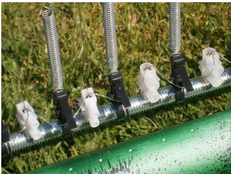
Figure 5 – A section of a finished rod. Note how the connecting wires are looped under the tie-wrap tails. Note both the tie-wraps and connectors are too tight to the rod in this example. Note the routing of the connecting wire under the insulating tie-wraps. Photograph – Andrew Durham
